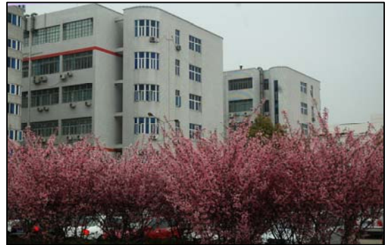
FCMS Bumping Facility – Shanghai, China
