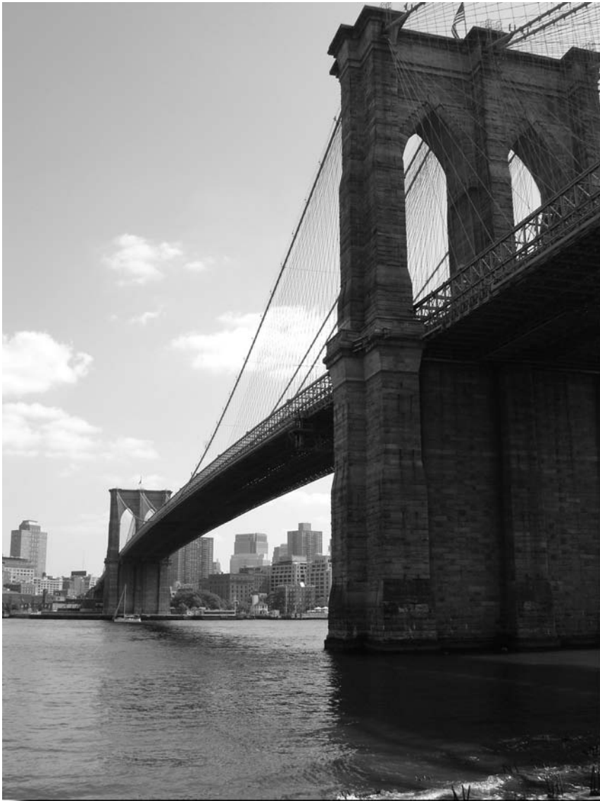
FIGURE 1-1: The Brooklyn Bridge from its base.
